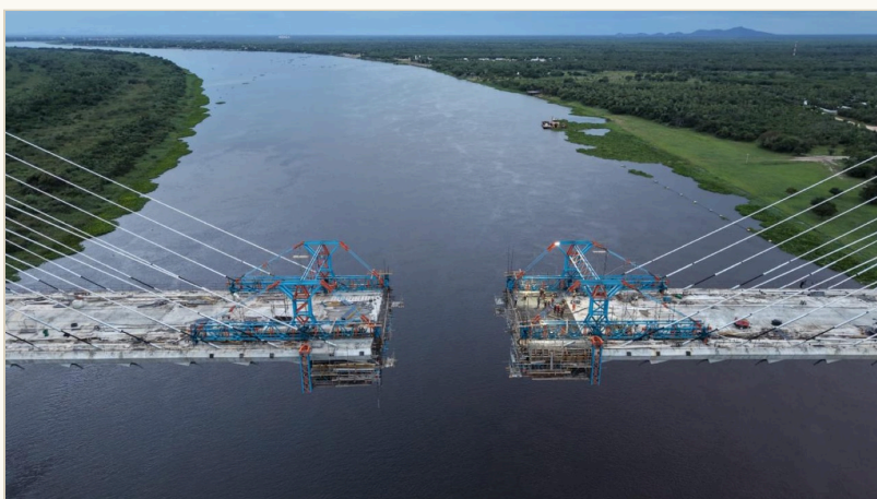
Bioceanic Corridor international bridge under construction (Jun 2026) — 55 km away. The driver of capital appreciation.
